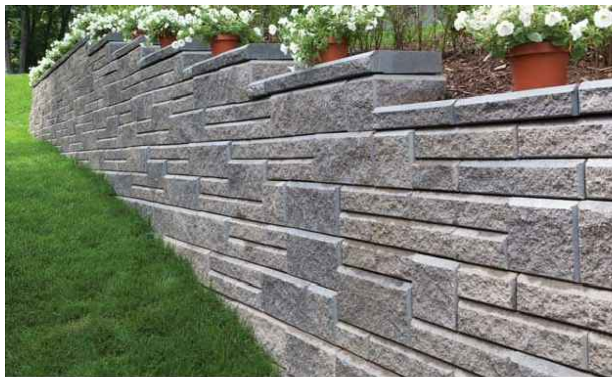
COLOR: GRAY BLEND FINISH: ALLAN BLOCK ASHLAR BLEND PATTERN NOTE: LOCATED ON BLOCK 26 ON NORTH SIDE OF BUILDINGS
