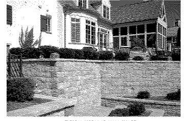
TYPICAL MODULAR WALL IMAGE GREY COLOR, CONCRETE BLOCK WITH WEATHERED ROCK TEXTURE CONCRETE BLOCK, 8" HIGH x RANDOM WIDTHS DESIGN BUILD MISE GEOMETRIC RETAINING WALL. BASIS OF DESIGN IS KEYSTONE CENTURY SERIES OR EQUIVALENT.
